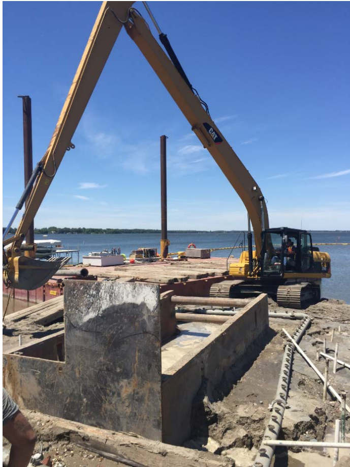
Dewatering at shore
