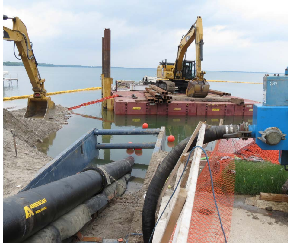
Initial setup for installation of intake line
