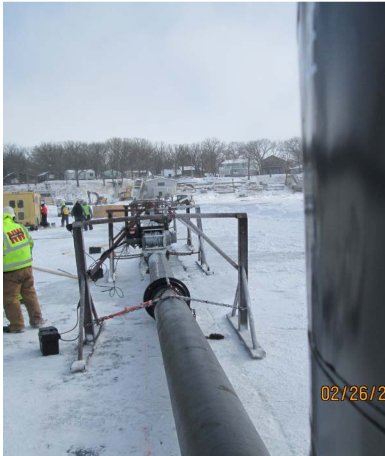
Laying out intake piping on frozen lake
