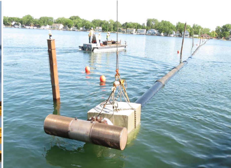
Installation of intake screen
