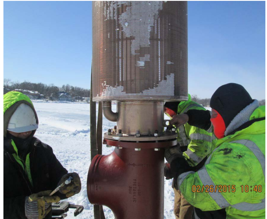
Assembling new 16-inch intake screen
