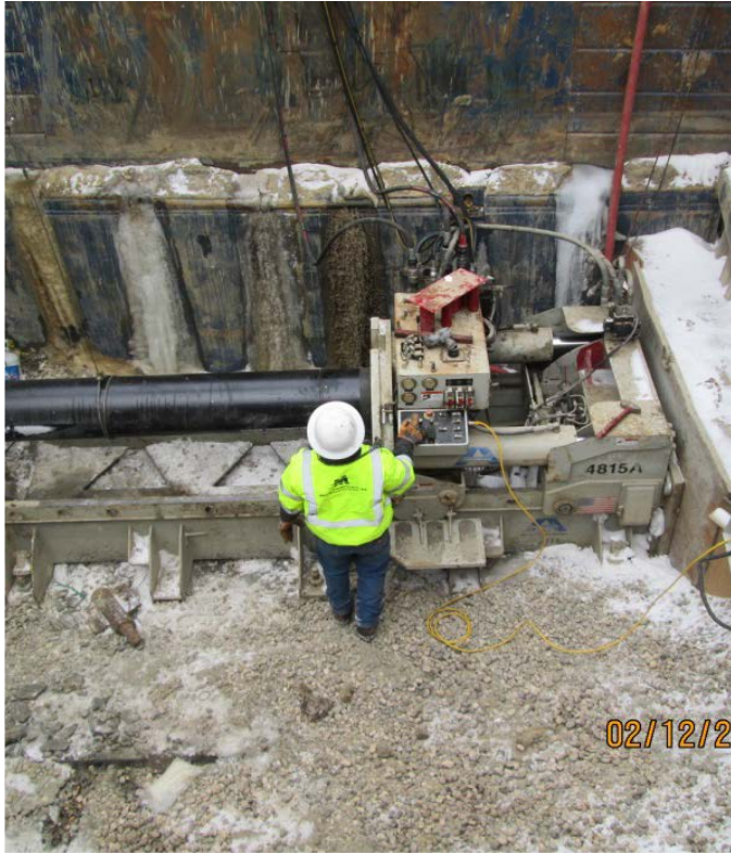
Installing the new 16-inch pipe from shore
