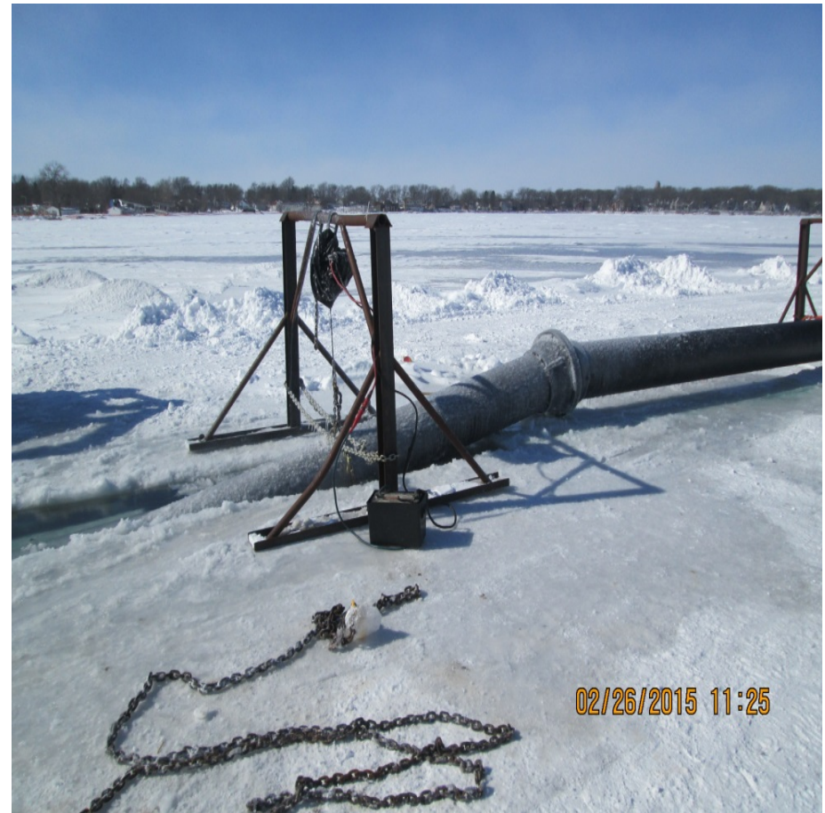
Lowering intake pipe through ice
